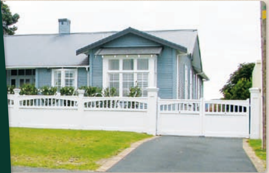
The Sunbury is a very solid design with ex100 x 25 TG&V at the bottom and 40 x 40mm vertical battens in the top. The gates above are hung on Ex300x300 Manhattan feature posts with matching Sunbury fence panels.
